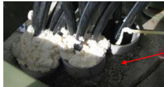
Apply expanding foam in between all cables to form a complete seal.
